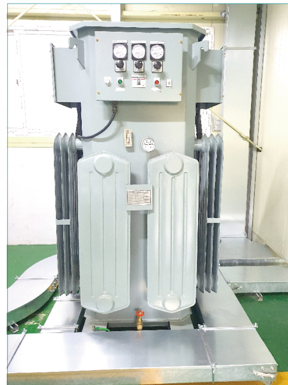
IVR [Isolating Voltage Regulator] 200KVA
